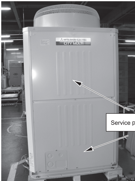
1. Remove both the top and bottom service panels (front panels).
