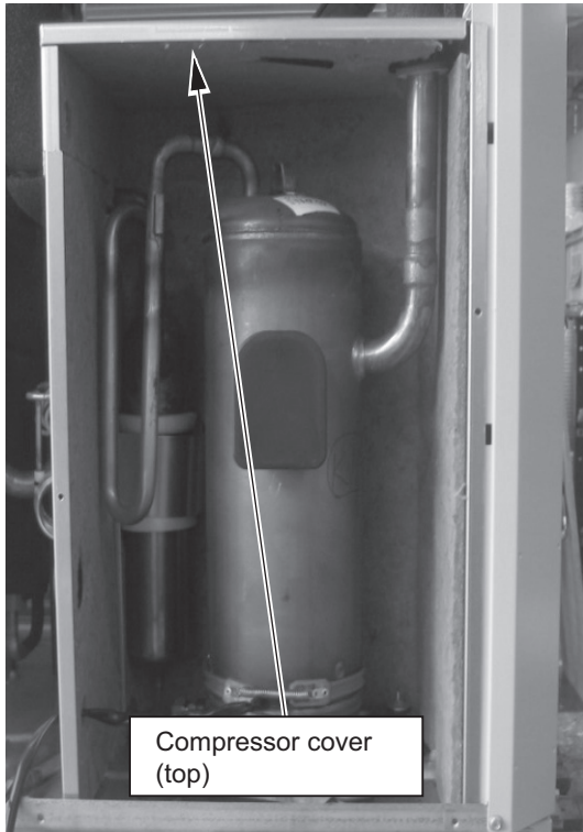
4. Remove the compressor cover (top).
